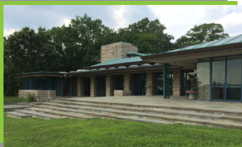
Rear terrace of the Corbett residence.
