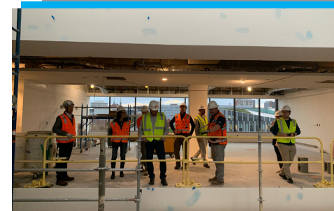
Skanska presenting a construction tour at University of Cincinnati
